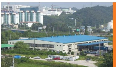
—• Head Office and Factory - 1
